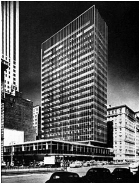
At the apex of the development of the Modern style are buildings like the Lever House office building in Manhattan (1952). They are, basically, what you can see: horizontal layers—beams and floor slabs—tied together visually and structurally by vertical column lines. If you could see the bare skeleton of the structure, the apparent insubstantiality of the materials would be revealed. Such is the efficiency and economy of Modern architecture.
